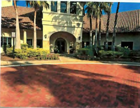
PHOTO 7 Clubhouse frontage documented during focused office and clubhouse detail work.
