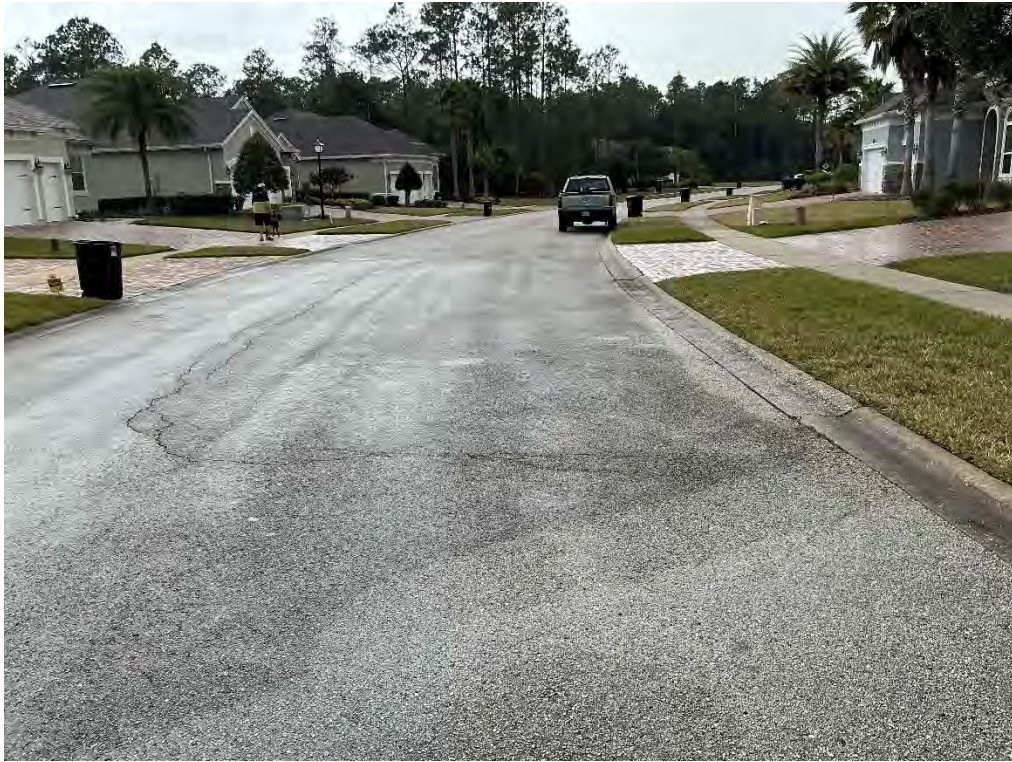
Photo 5801: About 15' wide of roadway depressed, View Westward.
