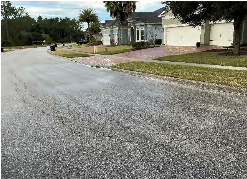
Photo 5807: About 46' length of roadway depressed, View Westward.
