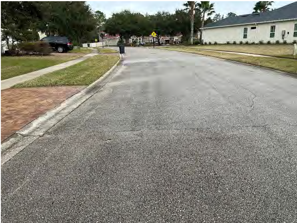
Photo 5799: About 15' wide of roadway depressed, View Eastward.
