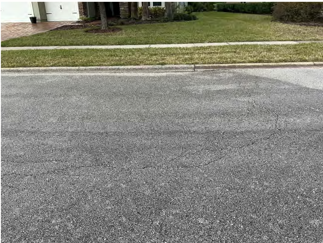
Photo 5797: Roadway depression at east end.
