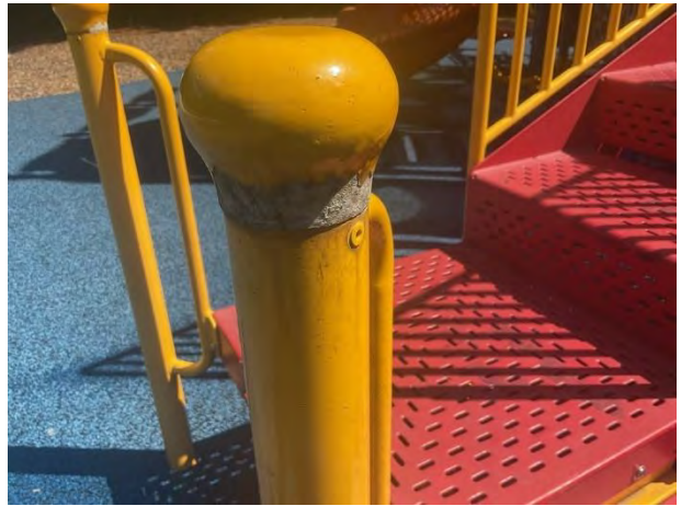
Equipment finish deterioration
