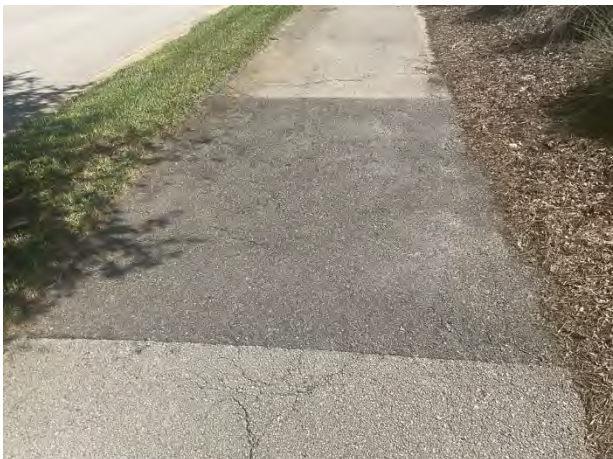
Asphalt pavement walking path previous repair
