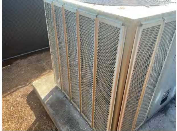
Split system condensing unit cabinet rust
