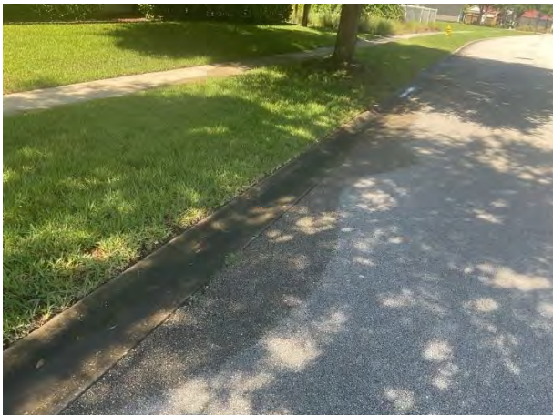
Concrete gutter
