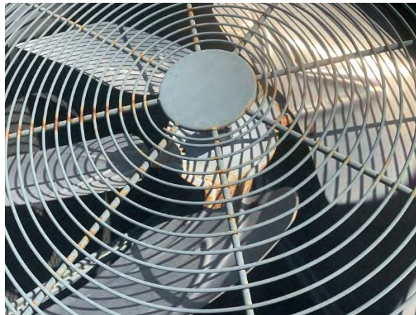
Split system condensing unit fan rust
