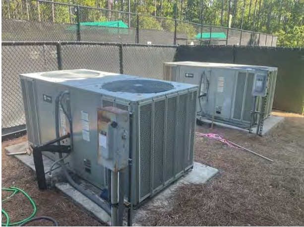
Split system condensing units
