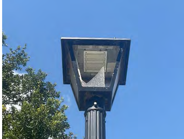
Damaged light pole and fixture
