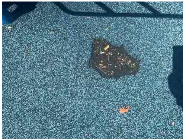
Safety surface depletion
