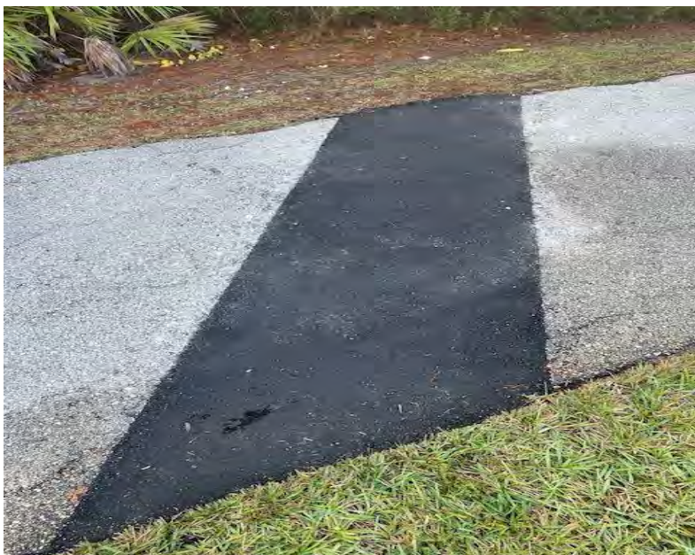
Cracked asphalt repaired along Ensenada
