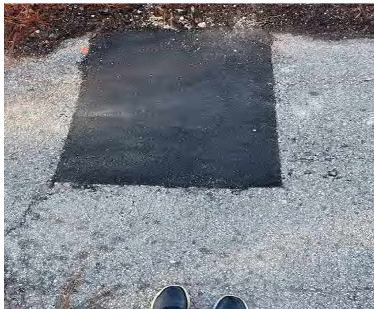
Cracked asphalt repaired along Ensenada
