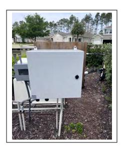
Installing metal lock boxes over the Smart Controllers.
