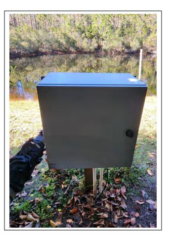
Installing metal lock boxes over the Smart Controllers.
